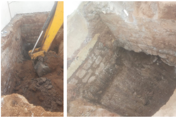
THE 10 FT DEEP PITS FOR FOOTINGS
