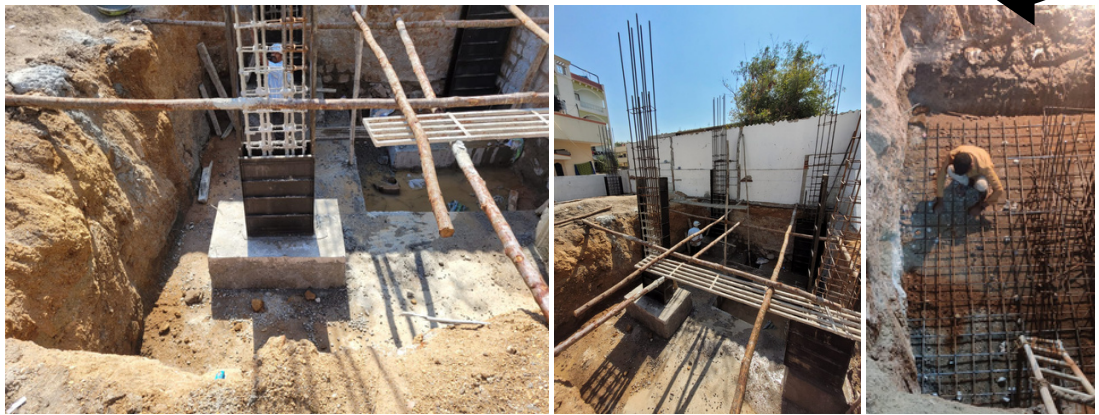
FOOTING BASE STEEL REINFORCEMENT, M25 READY MIX CONCRETE
